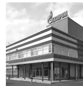
СК «Газпром Прометей» Construction Company "Gazprom Prometheus"
