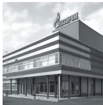
СК «Газпром Прометей» Construction Company "Gazprom Prometheus"
